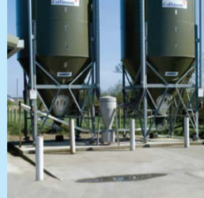
Empty and clean out bulk bins and connecting pipes
